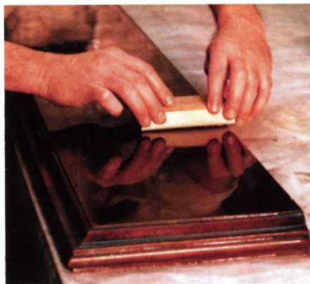
Photo 4 — Apply fresh mineral spirits, scrubbing with 220 grit sandpaper.
